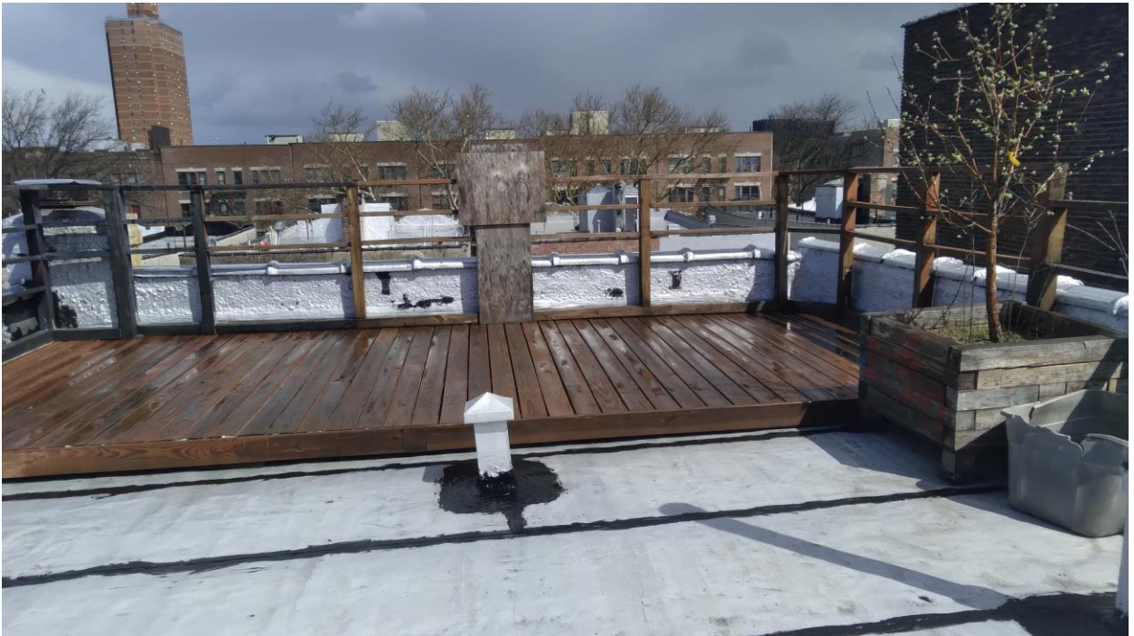
Back Portion Of Roof Deck
